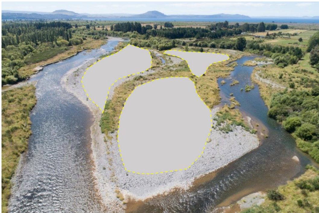
Figure 4: Island adjacent Kohineheke Reserve. Grey: Built up areas requiring lowering to annual average flow level.
