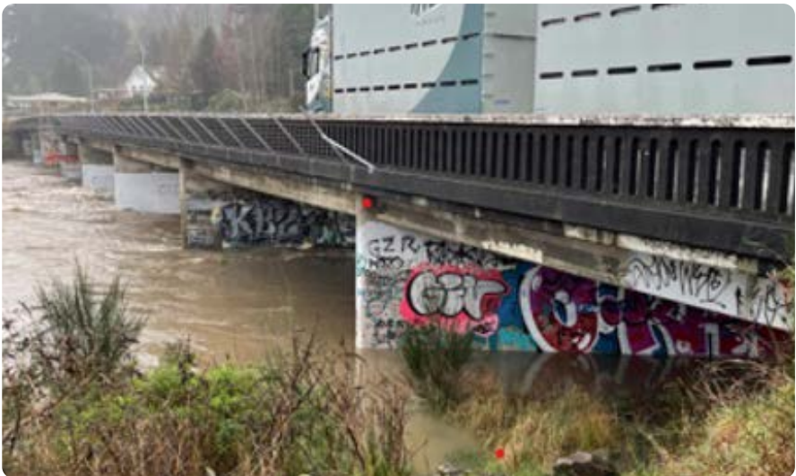
Tongariro River Bridge SH1.
