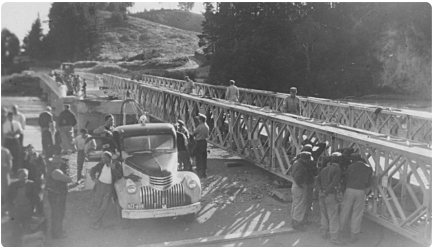
Temporary Bailey Bridge repair.
