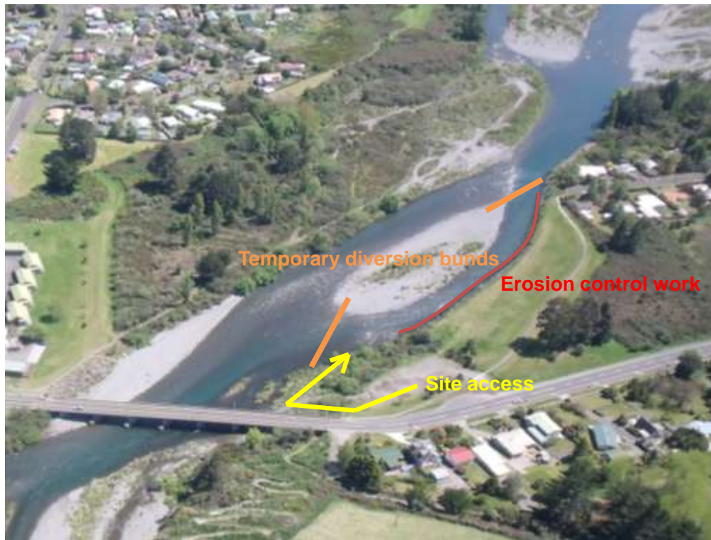
Fig 3. Access and work site description
