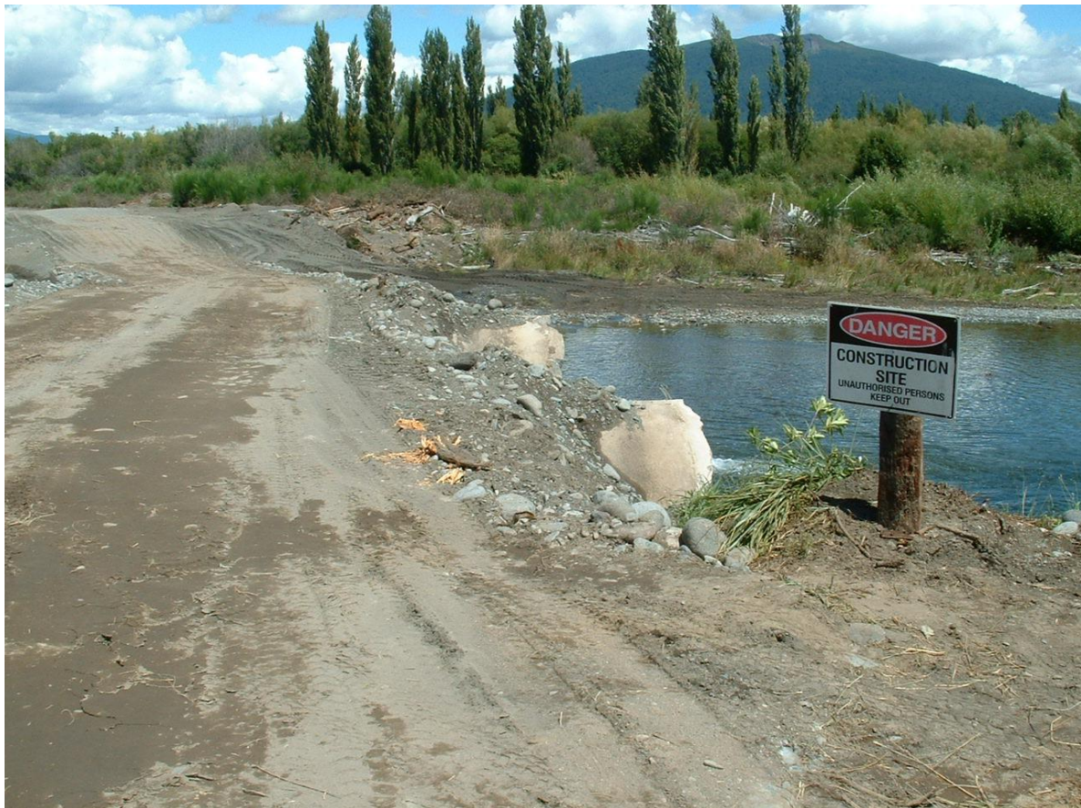
Figure 5: Example causeway to access gravel island. A causeway is considered low impact. Machinery can enter/exit avoiding disturbance of the bed and fish passage is maintained.
