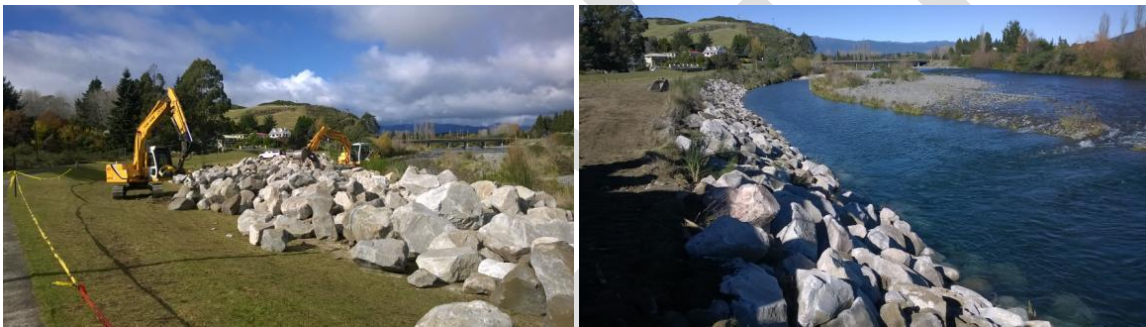
Figure 3 Works during 2013/14 rip rap top-up
