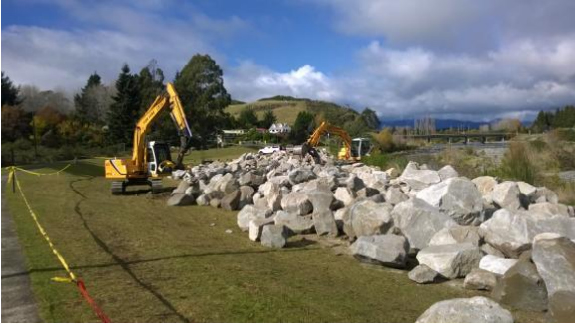
Figure 3 Works during 2013/14 rip rap top-up.
