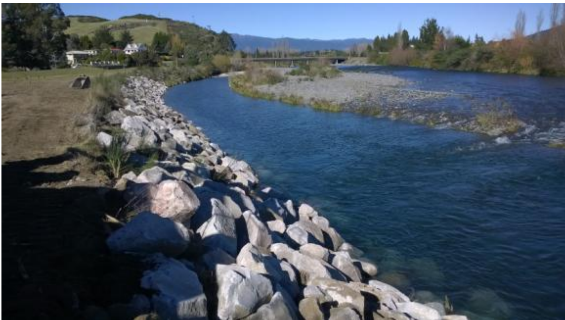
Figure 4 Herekieke St erosion protection after Rip Rap top up.
